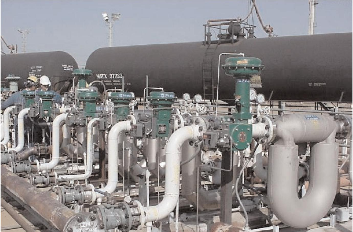
Micro Motion ELITE CMF300 meters on gasoline blending system in California
