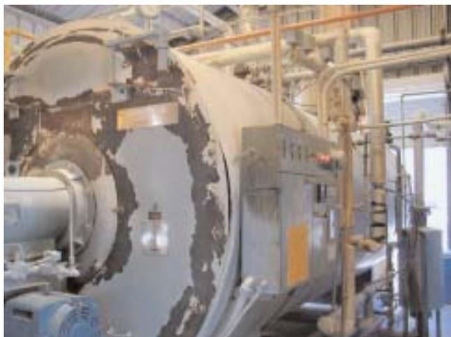
*The McIntyre Ga. facility's process steam boilers use as much as 20,000 cu ft per hour natural gas.*
