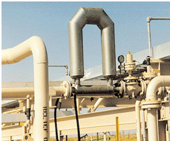
*The Micro Motion flowmeter performs accurately over a wide flow range, unlike the utility's rotary meter.*
