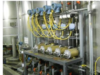
ELITE CMFS015 meters for charging polymer to aging tanks. These fractional sized meters provided best performance balancing accuracy and pressure drop.
