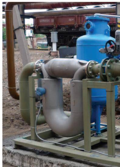
Micro Motion Coriolis meter measuring fuel oil.
