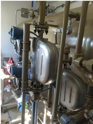
Micro Motion F-Series meters installed in well site gas allocation
