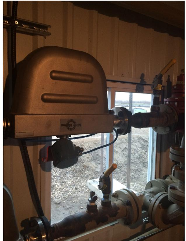
F200 meters in wet gas application for both high and low pressure lines off a heater-treater
