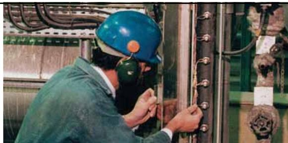
*The fault tolerant design of the Hydrastep continues to operate even if the circuit fails*
