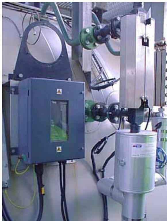
Figure 1 Hydrastep installation
