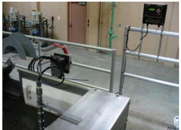
Figure 1: Gravity belt thickener
