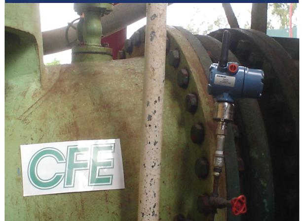
*Rosemount® wireless transmitters are used by CFE to receive key flow, pressure, and temperature measurements which are used to determine unit heat rates and equipment efficiency.*
