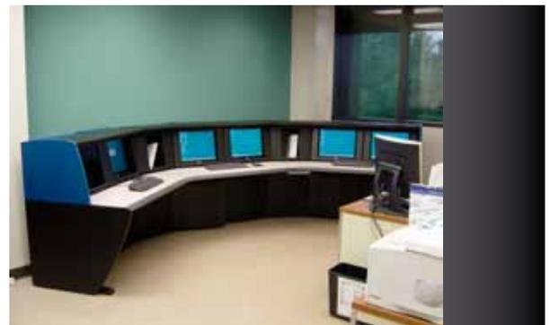
*Dairyland's J.P. Madgett Ovation Simulator mimics the control room layout to provide realistic training conditions for the plant operators.*
