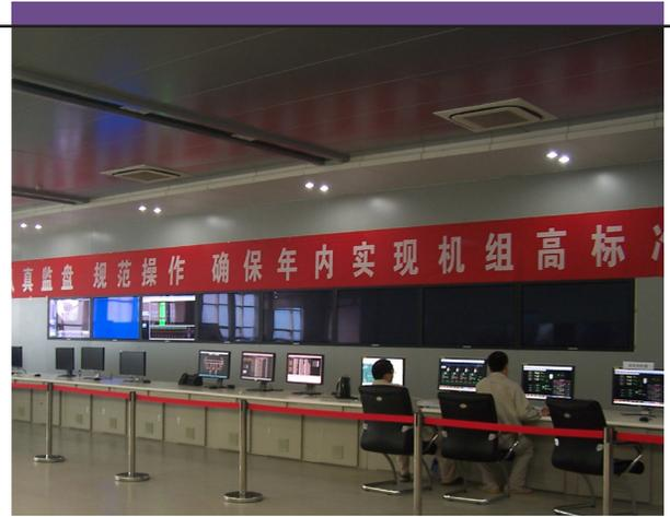
*The Pingdingshan control room uses state-of-the-art Ovation technology proven in 1000-MW ultra-supercritical units.*
