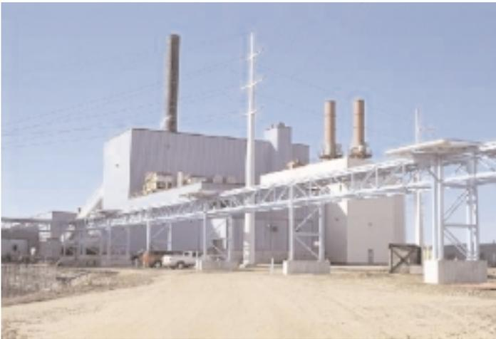
*Exterior, Rapids Energy Center cogeneration plant. Steam at 400, 150, and 50 psi is piped underground (directly below pipe bridge in the foreground) to the UPM Blandin paper mill unseen to the right.*
