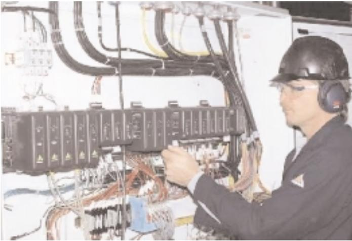
*DeltaV controller in a field cabinet adjacent to one of two new packaged gas boilers.*
