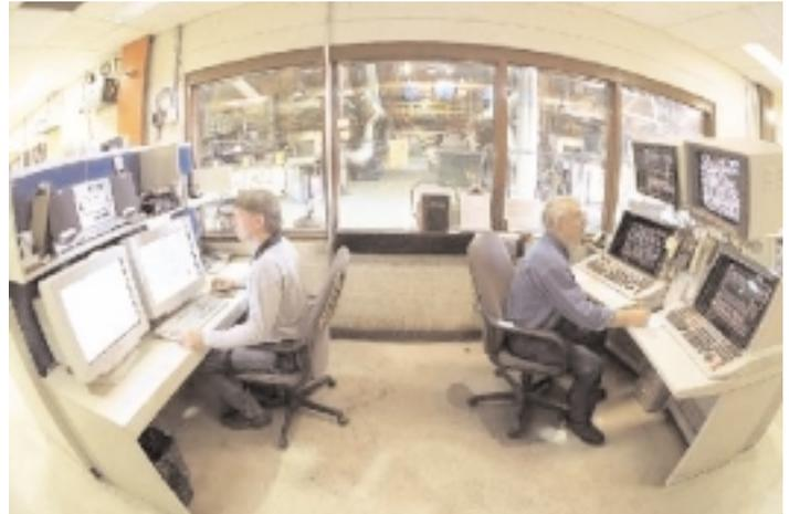
*On the left is the dual-screen DeltaV PC operator workstation for the new gas boilers, manned here by Mac Bonham, Station I&L; on the right is the existing PROVOX DCS operator console manned by Ray Nellis, Cogeneration Plant Operator.*
