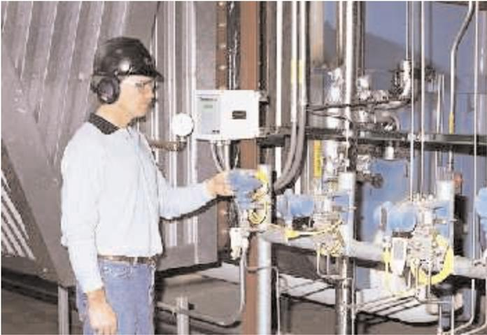
*Bonham at an instrumentation stand for Rosemount fieldbus transmitters adjacent to one of the package boilers.*
