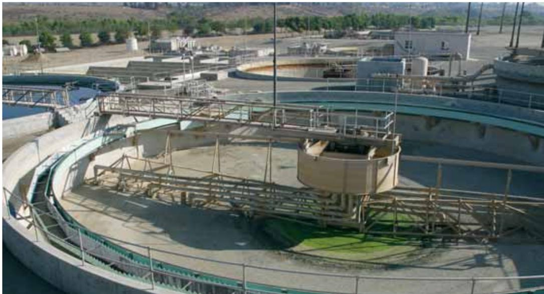
basin to remove up to 85 per cent of the remaining organic material. Dissolved oxygen (DO) is added to the aeration basin to provide oxygen to aerobic microorganisms so they can successfully turn organic wastes into inorganic byproducts, specifically carbon dioxide, and water. Maintaining an environment conducive to keeping these microorganisms alive and most productive is a critical job. If the DO
