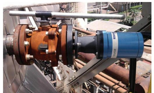
analyzers that are placed just ahead of the electrostatic precipitator in order to ensure that flue gases flowing through the precipitator have a low level of combustibles (CO) and a sufficiently high level of O<sub>2</sub>.
