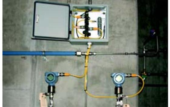
*Two Rosemount 3051S pressure transmitters connected to an Interlink BT brick.*
