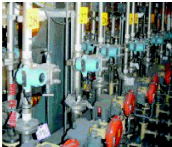
*3051SFP Integral Orifice Flowmeter
