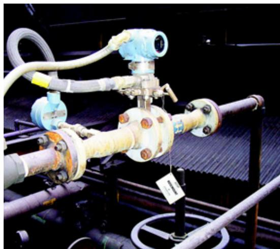
*3095MFC Compact Orifice Mass Flow Meter installed two pipe diameters downstream from multiple 90-degree elbows*
