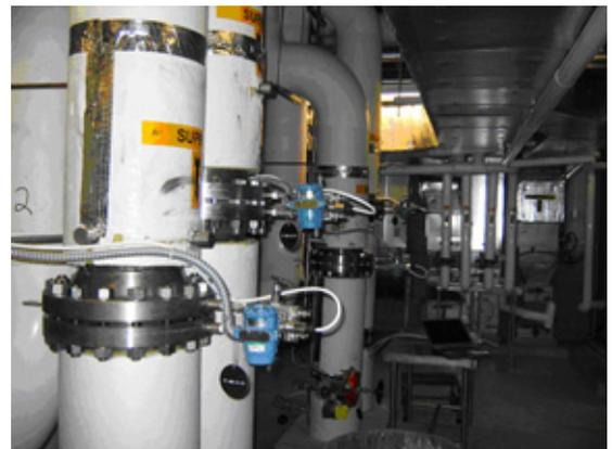
Figure 1. Conditioning Orifice Mass Flow Meter (1595 conditioning orifice plate with 3095 multivariable transmitter)
