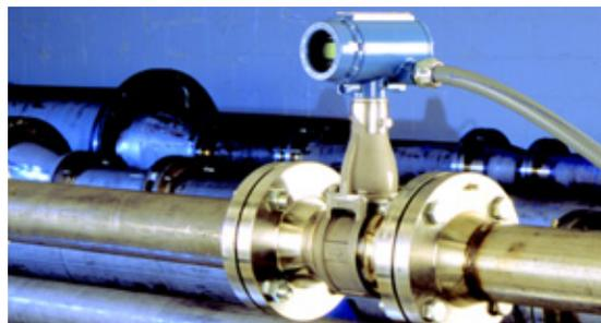
*The Rosemount 8800 Vortex Flowmeter Installed*
