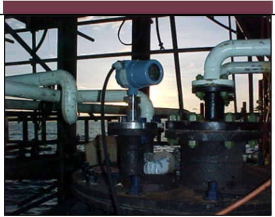
Rosemount 3302 is used to measure level and interface
