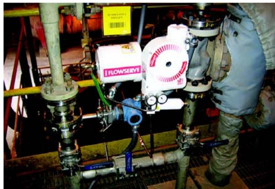
*Rosemount 3095MFC installation between multiple elbows, valves and limited straight pipe.*
