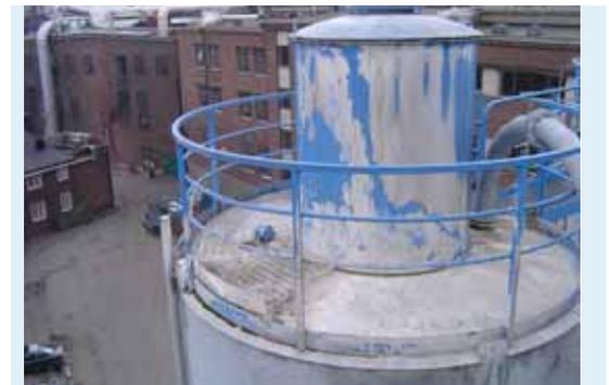
*The Rosemount 5300, with its advanced Guided Wave Radar features, reliably measures the lime levels, and is maintenance free even in the dusty environment of the lime silos.*
