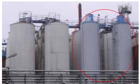
*The Quicklime silos, pictured in the front on the right, are used in the process of purifying the water used in production.*
