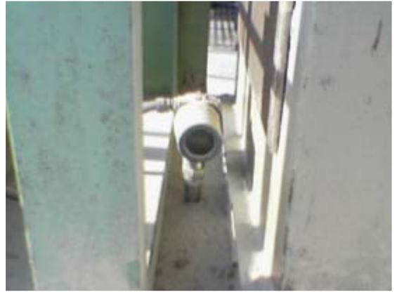
*The Rosemount 3300 was installed in the center of the silo, allowing it to reach well into the conical bottom.*
