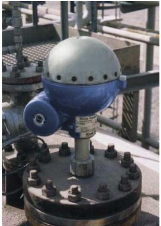
*The Rosemount 5600 Radar Level transmitter is mounted on the flange on the tank roof.*
