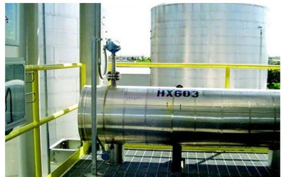
*A Rosemount 5300 with a HTHP single probe was installed directly into the glycerin reboiler*
