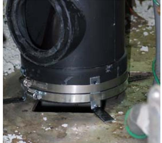
*During the temporary test installation the Rosemount 5401 was suspended over an existing tank opening.*
