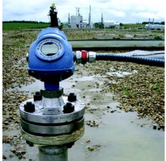
*The Rosemount 5400 was mounted on a stilling well shell. The antenna was trimmed to fit the smaller pipe inside*
