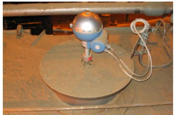
*The Rosemount 5600 is installed near the corner of the silo.*
