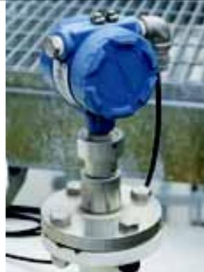
*Rosemount 3300 Guided Wave Radar Installed*
