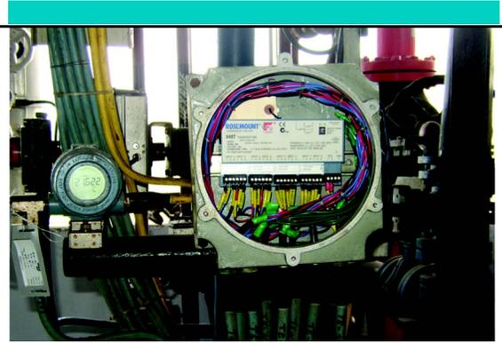
*A Rosemount 3244 MV and 848T installed in the field.*
