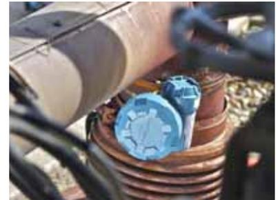
*Acoustic noise detected on the safety relief valve of an economizer alerted operators to a potential problem that risked a plant trip.*
