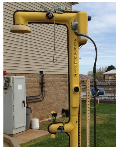
A 702 Wireless Discrete transmitter with TopWorx GO Switches communicate to a Smart Wireless gateway 1000 feet away to alert operators when the shower or eyewash station is activated.
