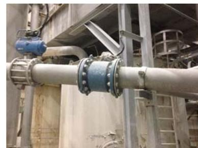
*Rosemount 8705 Magnetic Flowmeter installed in the most critical section of continuous machine feeding*
