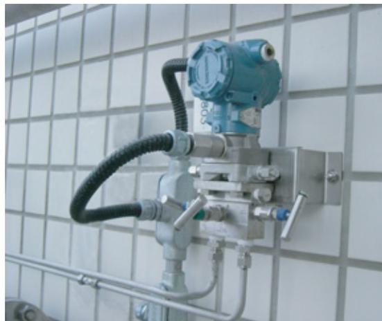
*Rosemount 3095 MultiVariable™ Mass Flow Transmitter.*
