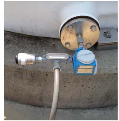
*Smart Wireless THUM Adapters provided cost effective replacement for deteriorated and failed wiring.*
