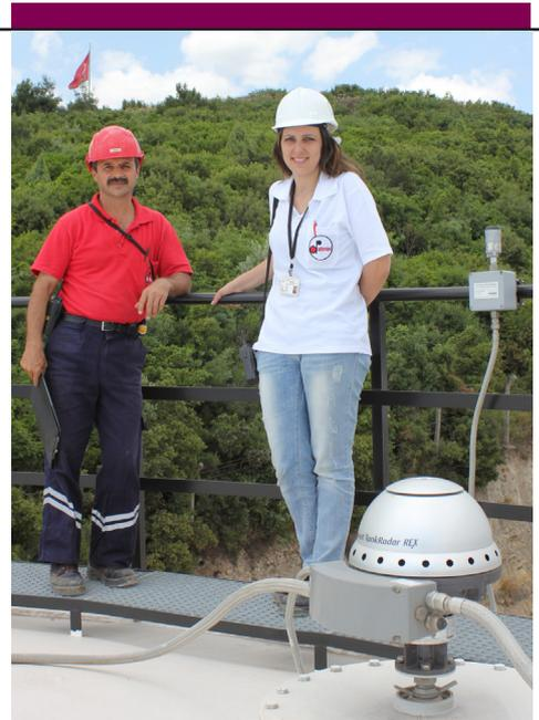
*When using automatic tank gauging there is no need for anyone to go on top of the tank. The risk is high, especially during a transfer, when the static electricity in the tank can be as much as 35.000 V. It is a great advantage to watch from a distance.*
