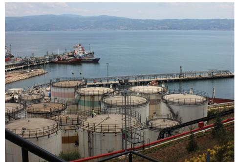
*Liquids are landed by tankers at the Altintel jetty, and further pumped into the storage tanks. 50-70 trucks are loaded daily, to provide Altintel's 2200 customers with their product blend.*
