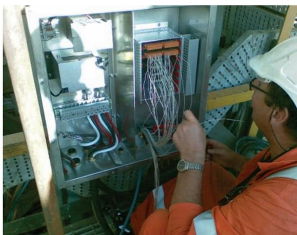
Figure 2: installed sensing pins with field cables and termination in an on-line instrument.
