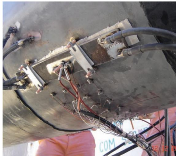
Figure 1: installation of FSM, non-intrusive monitoring in Brazil
