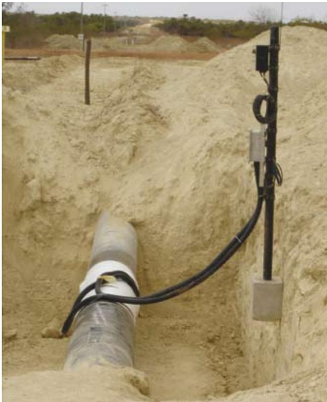
**Figure 2. An offline electric field signature system on an underground pipeline in Brazil.**
