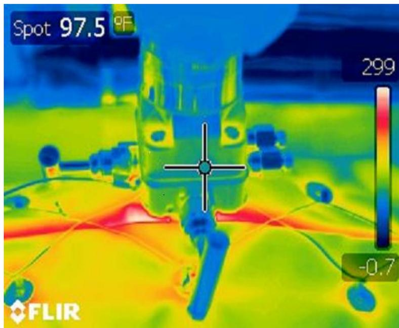
Figure 8 shows an example of a 1495 orifice plate installed on 250 °F (121 °C) saturated steam with a remote mounted transmitter. This installation has also been in operation since June 2008.
