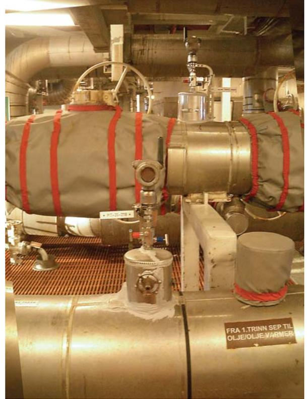
*The Rosemount Smart Wireless pressure transmitters are used to measure pressure drop over the platform heat exchangers.*
