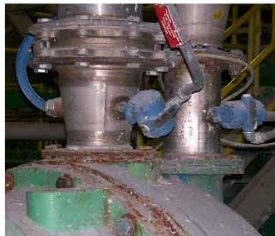
Figure 1. Installed Rosemount 1199 Gage Pressure Transmitter with Super Duplex 2507 material.
