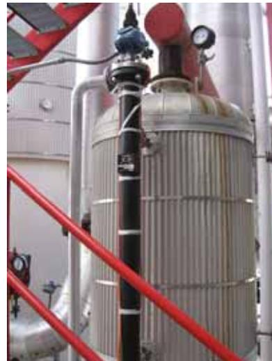
Figure 2: This is the 3-in. diameter Rosemount 9901 Chamber prior to adding insulation.
