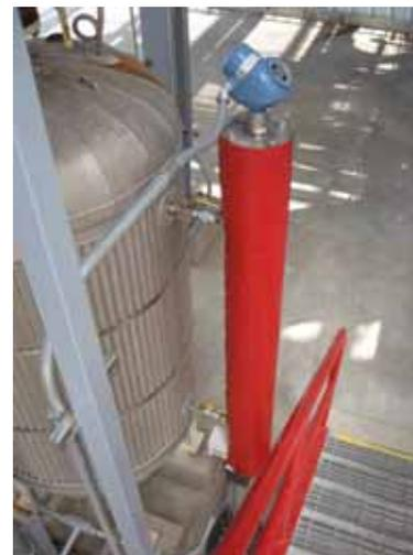
Figure 3: Rosemount 5301 (GWR) with Rosemount 9901 Chamber.
