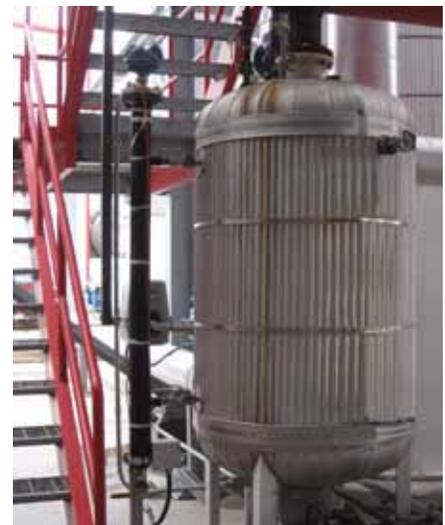
Figure 1: Rosemount 5301 Guided Wave Radars mounted on Rosemount 9901 chamber for condensate receiver level control.
