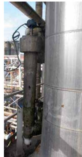
Figure 1. Rosemount 5301 with Diagnostic Suite used for monitoring abnormal process conditions.
