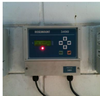
*Rosemount 3490 controller used for local display and alarms*
