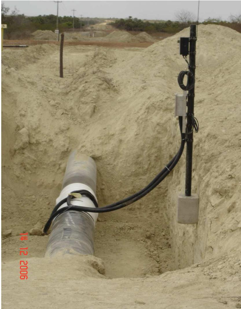
*The FSM matrix installed on an underground pipeline.*
