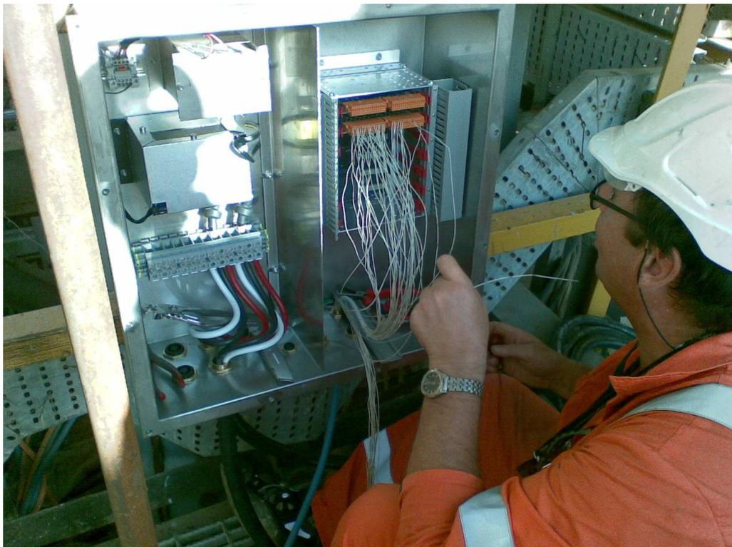
***Termination of the cables in the FSMLog instrument***
