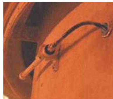
*A remote antenna on the center rotating shaft inside the sugar silo allows the wireless instruments to communicate with the Smart Wireless Gateway located outside each silo.*
