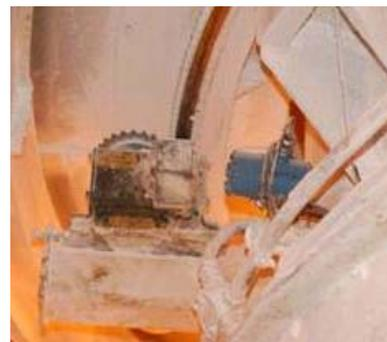
Four 648 (single point) Smart Wireless Temperature Transmitters were placed inside the silos to measure bearing temperatures and motor currents.
