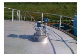
Figure 3.4: Manways are normally located near the tank wall which provides mechanical stability.
