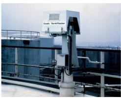
Figure 2.9: First high precision radar gauge installed in 1985 on a refinery tank.
