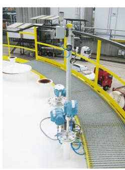
Figure 9.8: Antenna connected to tank devices.
