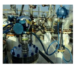
Figure 9.3: Tank redundancy is accomplished with dual tank gauges and separated communication layers - wired and wireless.
