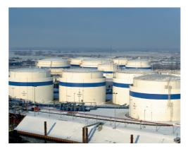
Storage tanks are often placed in clusters or tank farms. The tanks are atmospheric, pressurized or cryogenic.
