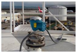
Figure 2.10: Modern radar level gauge on a fixed roof tank.
