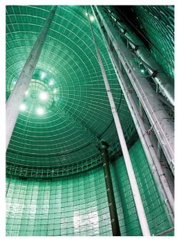
Picture 7.4: Full containment tank used for storing refrigerated liquified gas.
