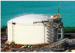
1.4: Cryogenic tank storing LNG at -162°C.
