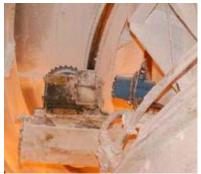
Four 648 (single point) Smart Wireless Temperature Transmitters were placed inside the silos to measure bearing temperatures and motor currents.
