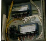
One 848T Wireless Temperature Transmitter can handle up to 4 inputs including 4-20mA, mV, Thermocouple, RTD, or ohm. The field hardened enclosures and intrinsically safe Power Module makes it ideal for this hazardous environment.
