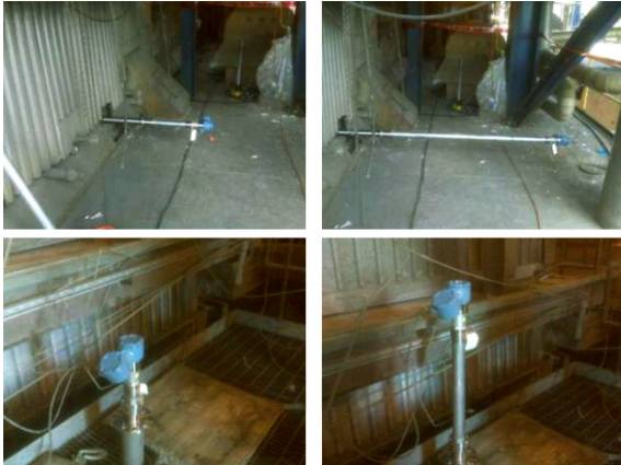
Figure 11 - Variable insertion O 2 probes in horizontal and vertical orientations.
