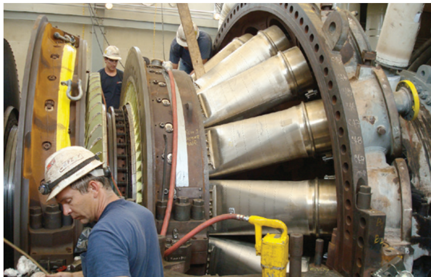
4. More durable transition pieces are visible as millwrights install combustion system
