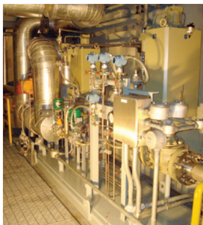
15. Fuel-gas valve skid (left) and water-injection system skid (right) were made in the US to meet schedule commitments
