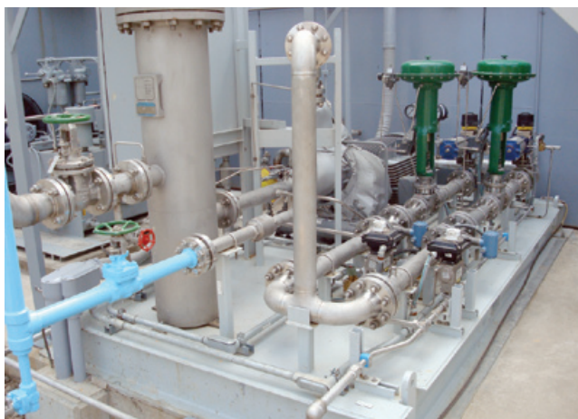
15. Fuel-gas valve skid (left) and water-injection system skid (right) were made in the US to meet schedule commitments
