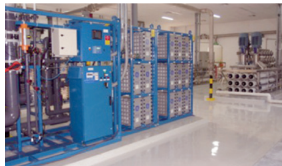
13. Raw water is pumped from a municipal aquifer to the pre-treatment system. Permeate from the RO unit at right in photo is polished by the EDI (electrodionization) system at left. Staff pride is evident from the level of cleanliness
