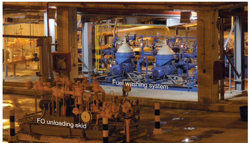
10, 11. Centrifuges for fuel washing are located inside fuel-treatment shed; one unloading station is in the foreground (left). Flow diagram gives details on the fuel treatment system (below)
